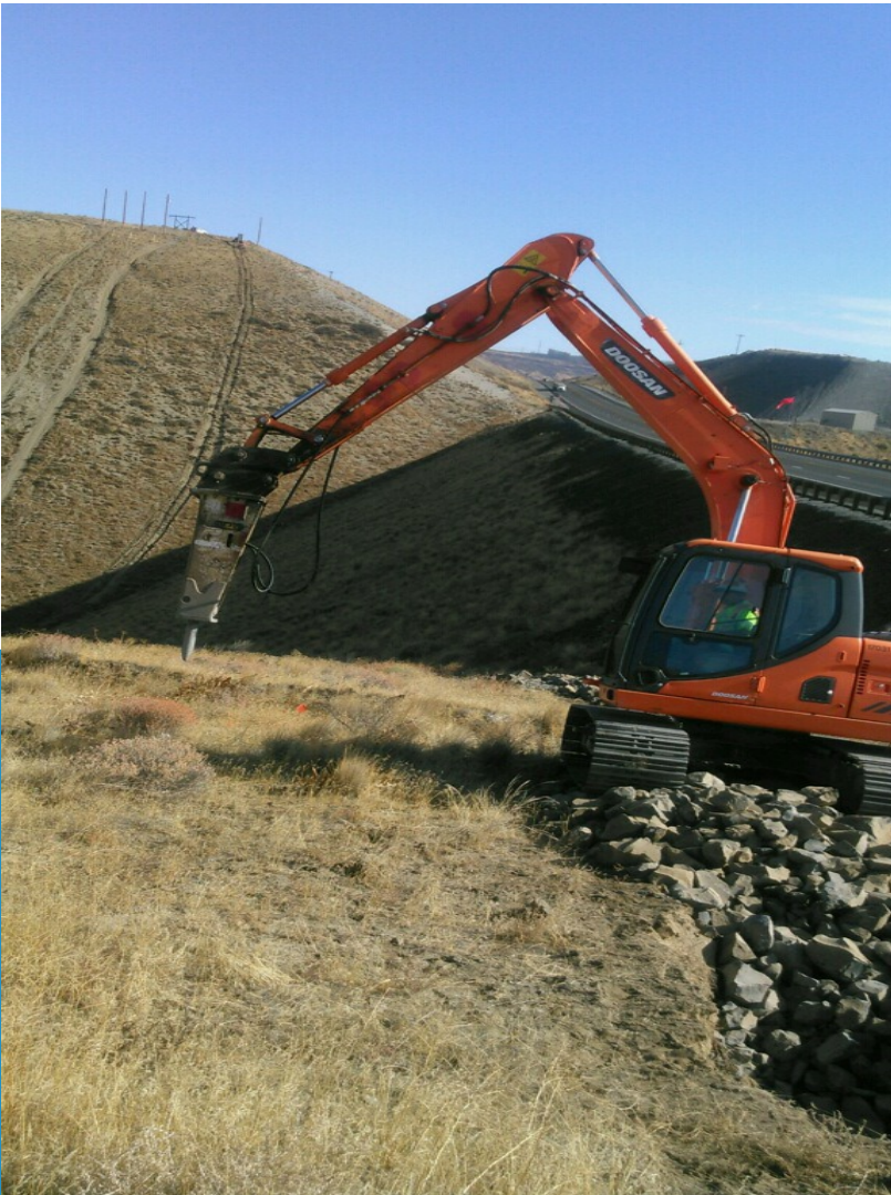
Excavator with rock hammer. Breaking rock for a fiber trench
