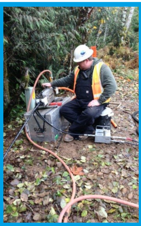
Fred Steinbach blowing 144 count fiber in, Gig Harbor Wa.
