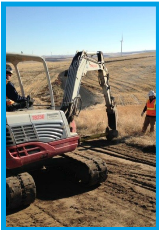
Tony Jensen operator with Roberto Hernandez; groundman performing cleanup after placing new conduit on Tucannon River Wind farm near Dayton, WA.
