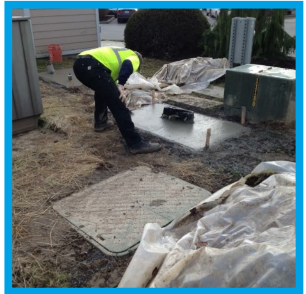
Bert Pegg finishing concrete on a cabinet site. On Lopez Island in Washington
