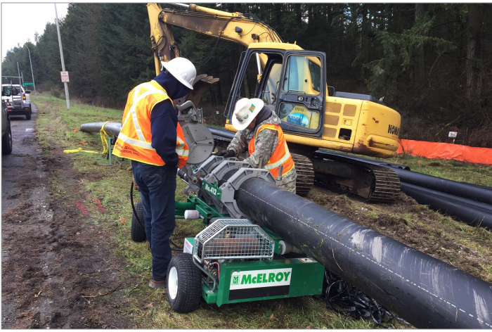
LEFT: RBC team members utilize a portable fusion machine to weld 40-foot lengths of 8-inch gas line. RIGHT: The 8-inch HDPE gas main was installed in trench with a "benching" technique for safety and better access. BELOW: Former Alaska governor Bill Walker stands with RBC CEO Dan Cook at the kickoff for the IGU project.
