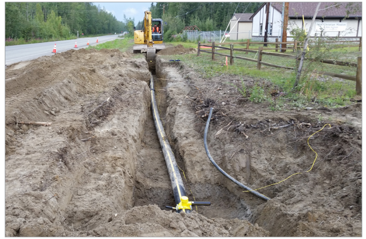
LEFT: RBC team members utilize a portable fusion machine to weld 40-foot lengths of 8-inch gas line. RIGHT: The 8-inch HDPE gas main was installed in trench with a "benching" technique for safety and better access. BELOW: Former Alaska governor Bill Walker stands with RBC CEO Dan Cook at the kickoff for the IGU project.
