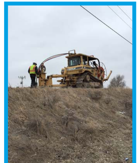
Plowing for new customer Viaero Wireless
