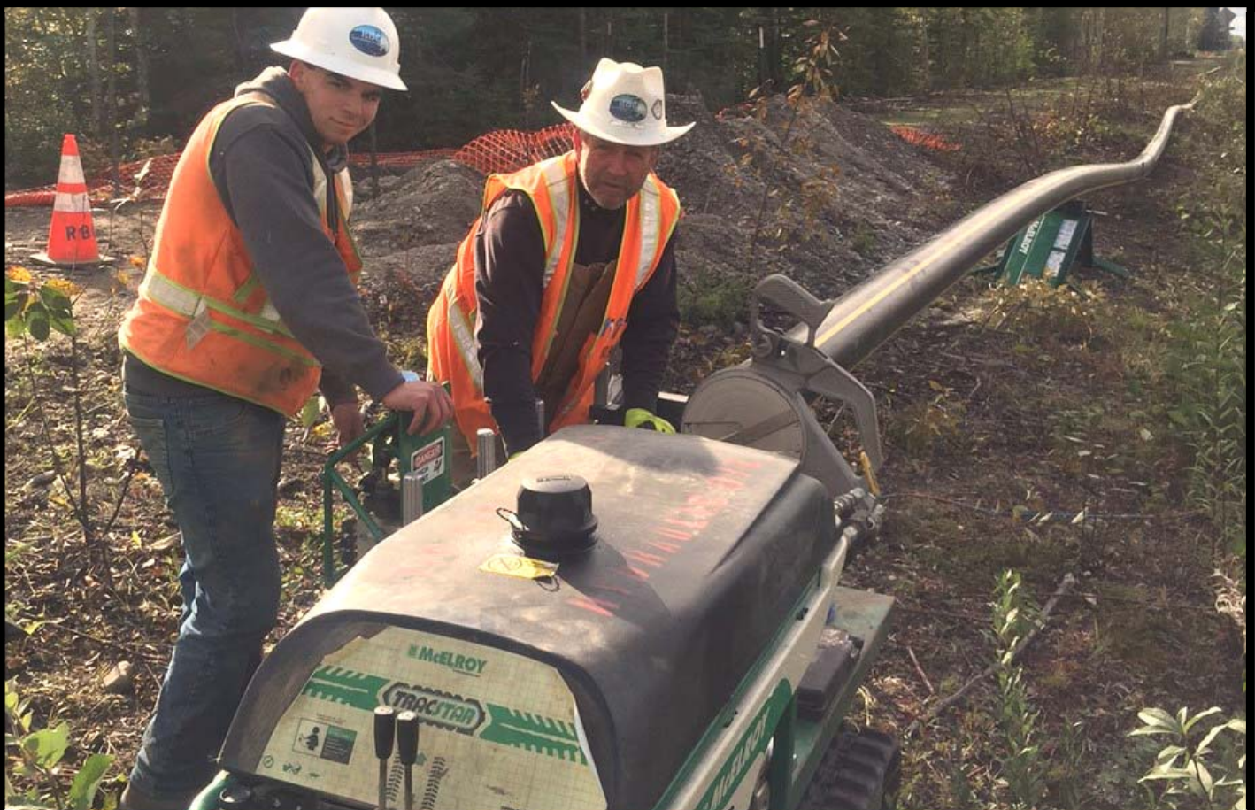
Ralph Griffin & Tyler Sepesi-Benson fusion 8" piece with a pulling eye to pull back a 800' bore in the morning
