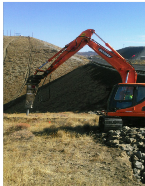
LEFT: A large crane is utilized to install a premanufactured fiber optic signal regeneration building. RIGHT: An excavator breaks through rock to make way for a fiber trench.
