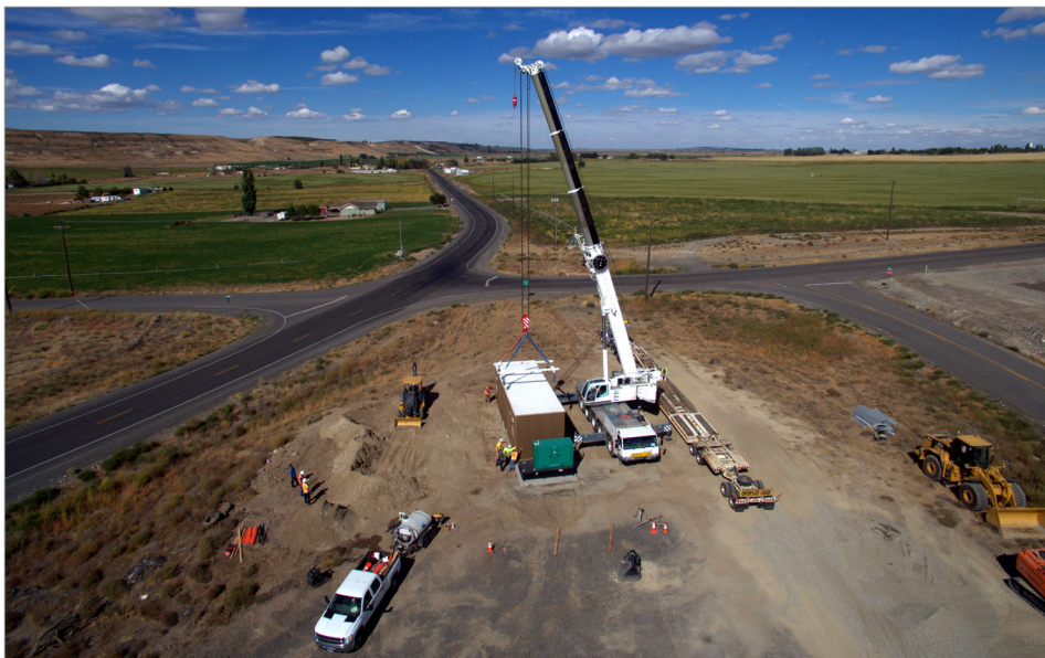
LEFT: A large crane is utilized to install a premanufactured fiber optic signal regeneration building. RIGHT: An excavator breaks through rock to make way for a fiber trench.
