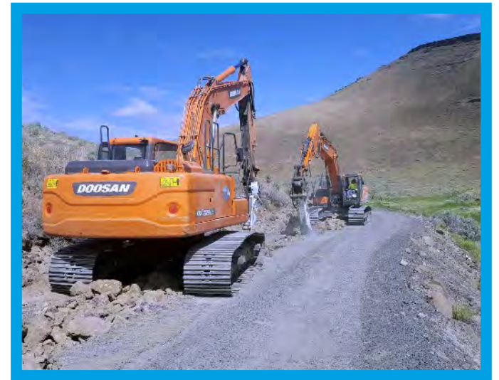
2-300 size excavator's with rock hammers
