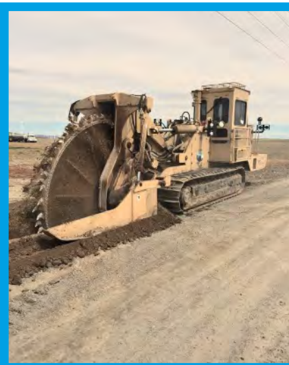
Dirt on top with 12" of rock in bottom
