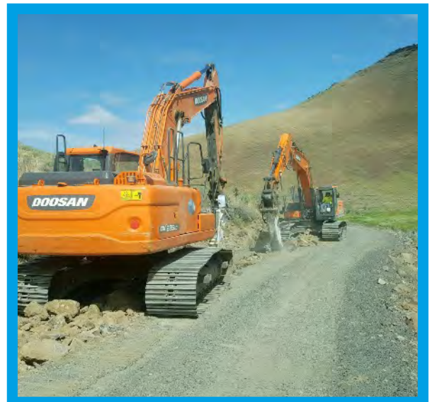
2-300 size excavator's with rock hammers breaking rock down the hill to the John Day River
