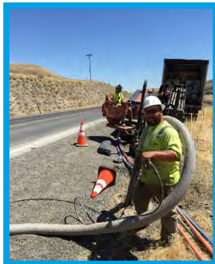
Pulling back a 500' shot under the rail road. Travis Smith operator on Drill and Ty Bain is groundsman/locator
