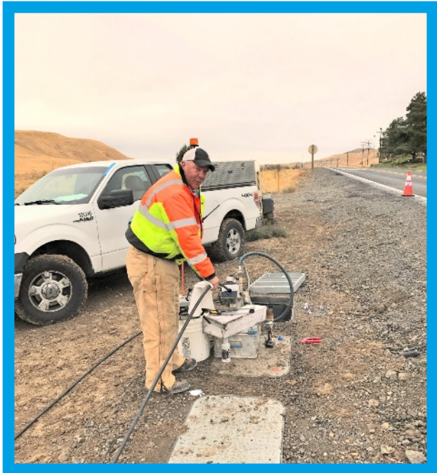
Sparky Murry - Blowing fiber near Arlington, OR
