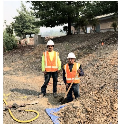
Potholing to place cable into Rogue Credit Union, Medford OR- Ramon Partida & Juan Aguilar
