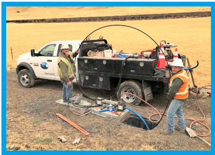
Andy Dirks & Larry Sterritt Blowing Fiber on large Zayo job Arlington, OR
