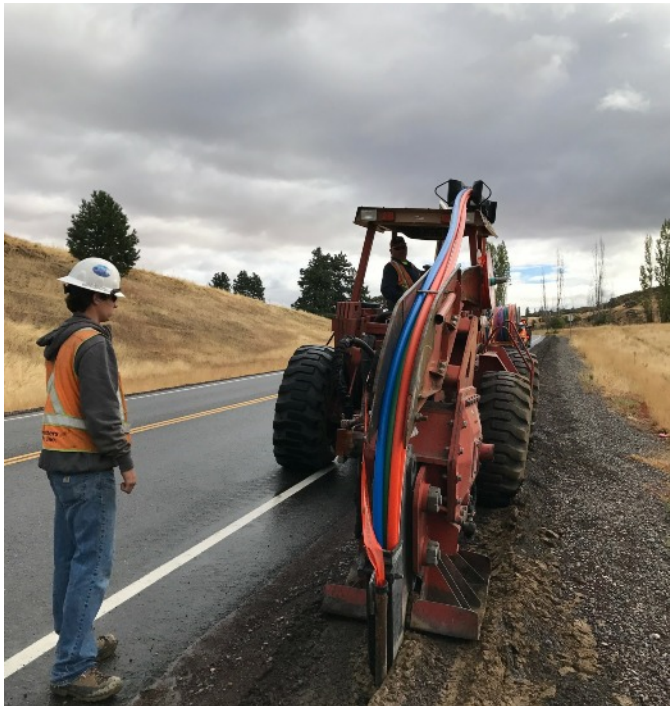
Plowing cable near The Dalles, OR w/RT185 plow Tim Cooper (operator), Chase McCall (groundsman)
