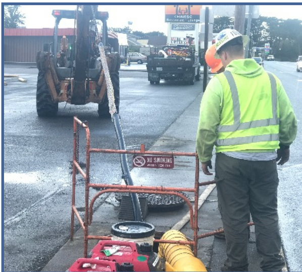
Pulling 1800 pair EMC Bandon OR Jessiup Hult
