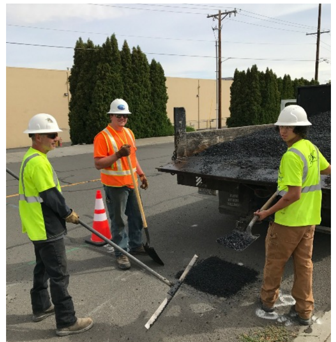
Paving Crew restoring asphalt in The Dalles, OR Owens Barnes, Dean Blasius & Alex Pedroza
