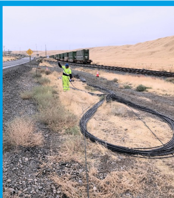
Chris Blayne - Walking out figure 8's for blowing fiber - Arlington, OR
