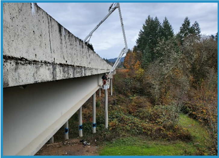
Tyler McMahan & Sam Farra placing conduit under Long Tom bridge. Noti OR
