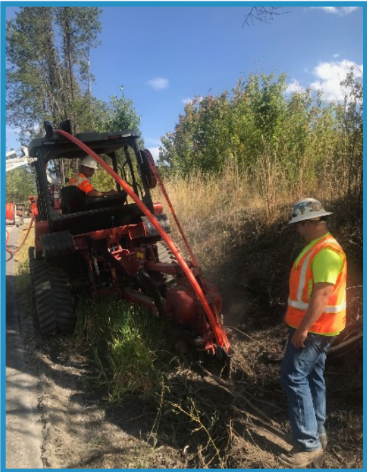
Jack Rains - equipment & Kendal McMillen - ground. Plowing conduit - Harrison ID
